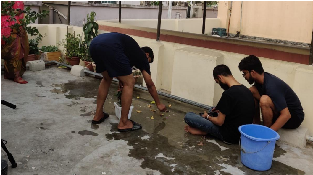
16.17 Description -ready to set.
